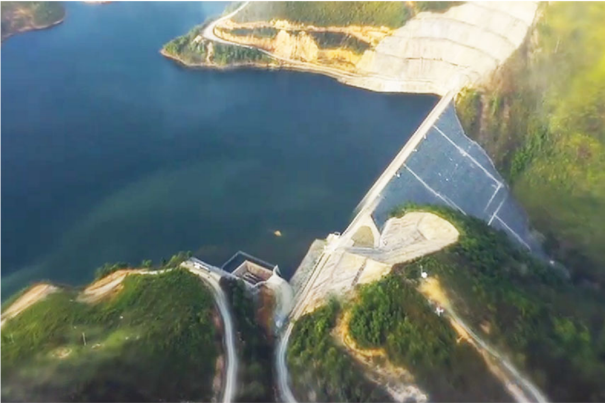
Nam Phay dam intake area view below:
