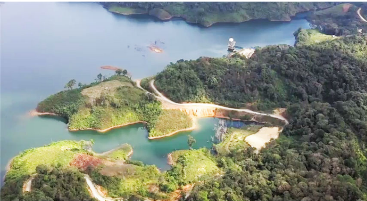
Nam Phay dam intake structure image below:
